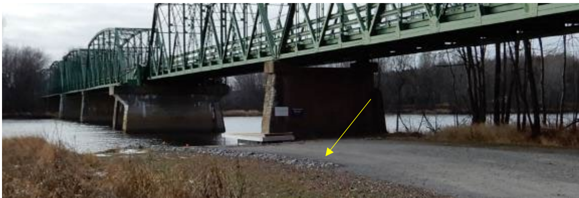
Figure 4-1 Enrochement existant
