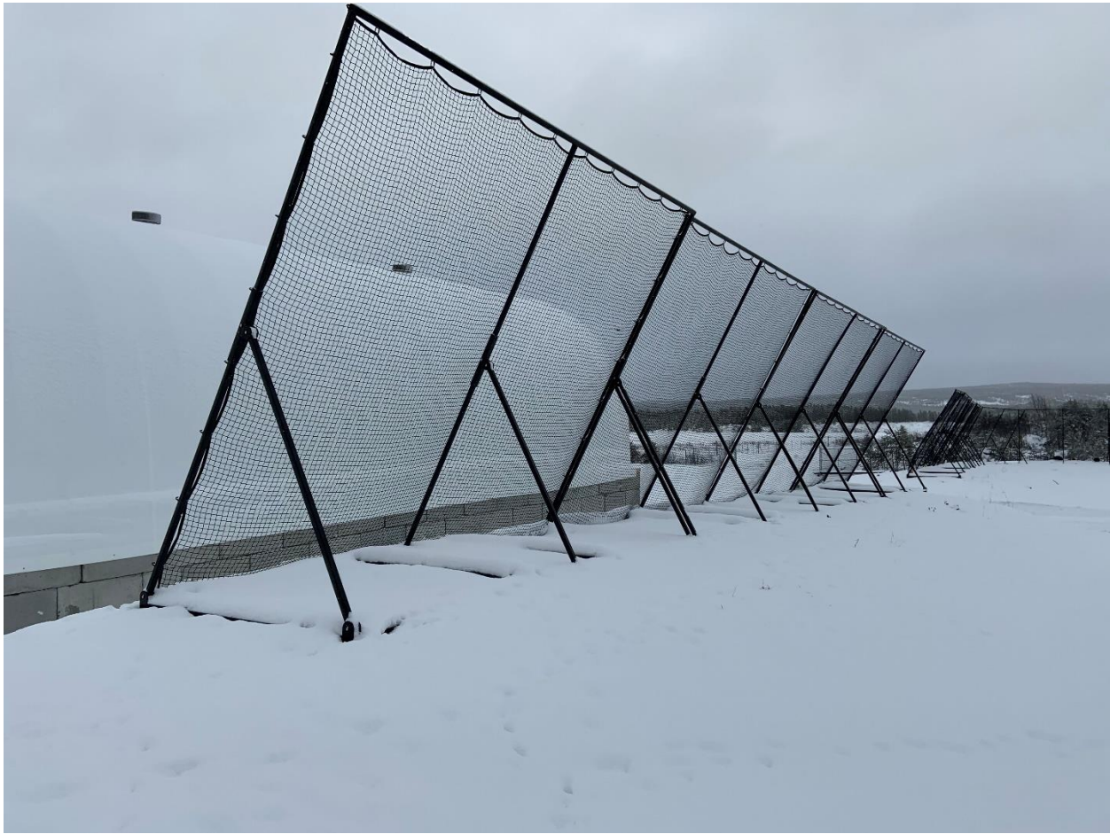
Figure 4 Capture nets currently used at the Nemaska landfill
