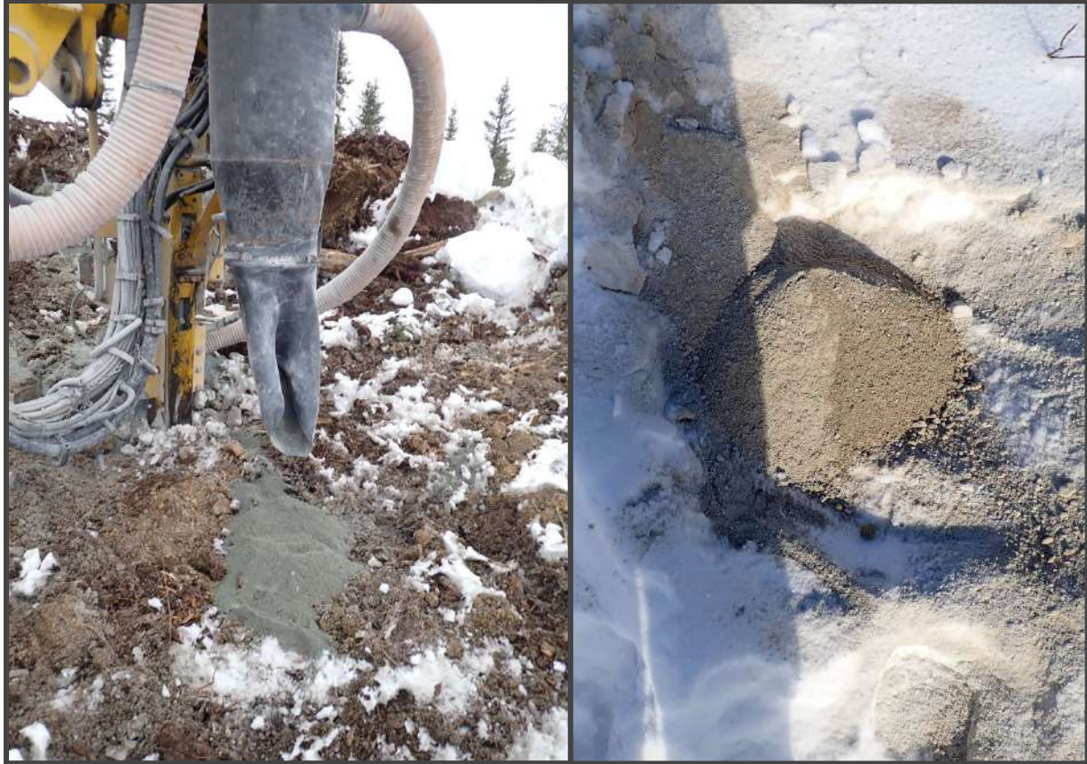
Figure 7: Photographs Showing Excavation Rock Drill Cuttings
