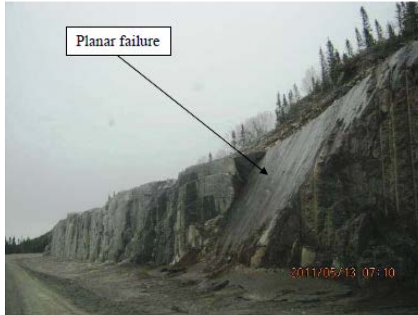
Figure 14-11: Planar Failure in a Rock Wall
