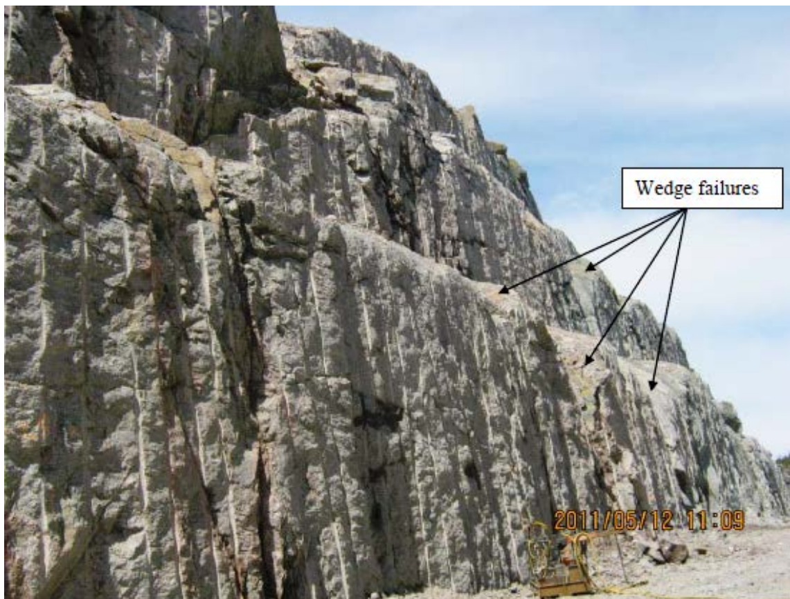
Figure 14-16: Pre-shearing Blast Over Three (3) 15-m High Benches
