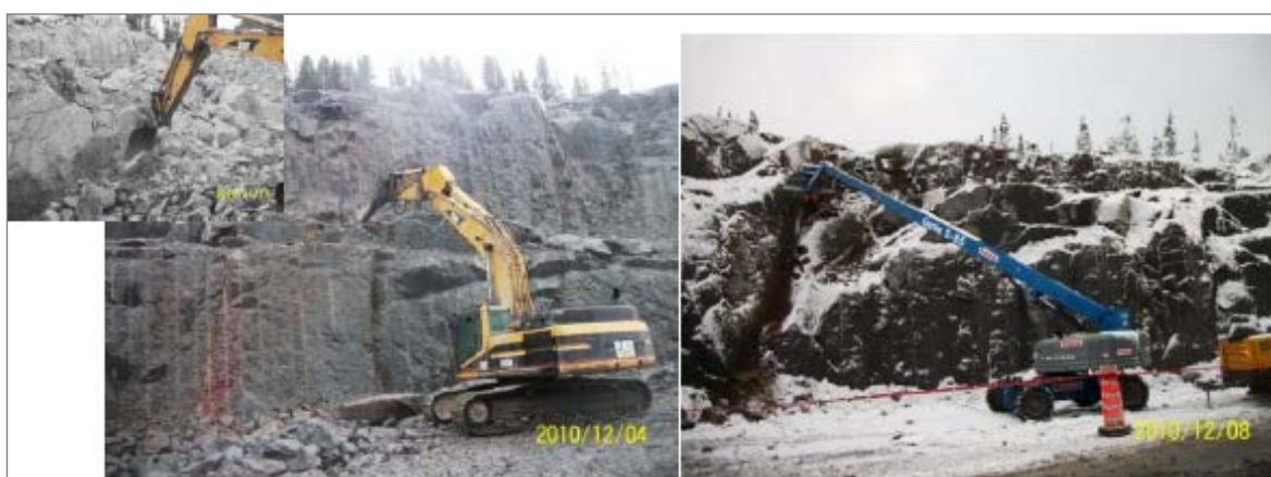
Figure 14-17: Scaling Methods; (left) Using an Excavator, (right) Using a Lift and Steel Bars to Pry Loose Rocks
