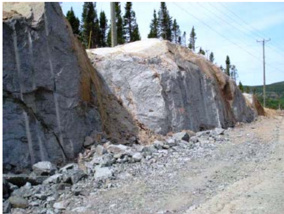
Figure 14-13: Wedge Failure Within Pre-shear of Rock Face
