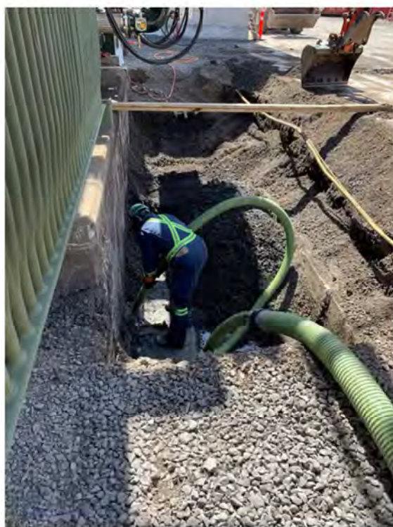
Photographie 4 Hydro-excavation – Excavation 1
