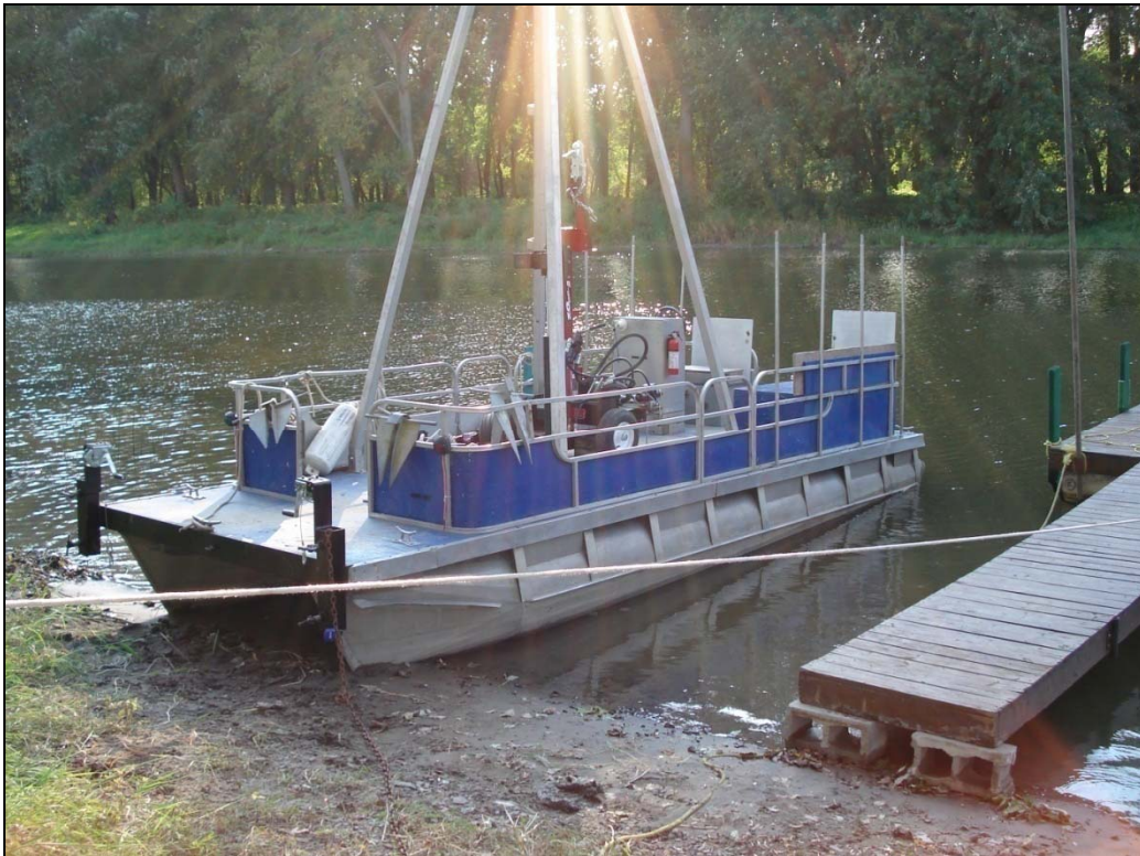
Figure 110: Barge for the Drill Rig
