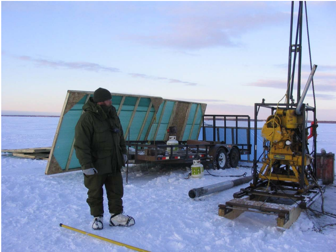
Figure 108: Sled Mounted Drill Rig with Shelby sampling tube to the left of the rig.
