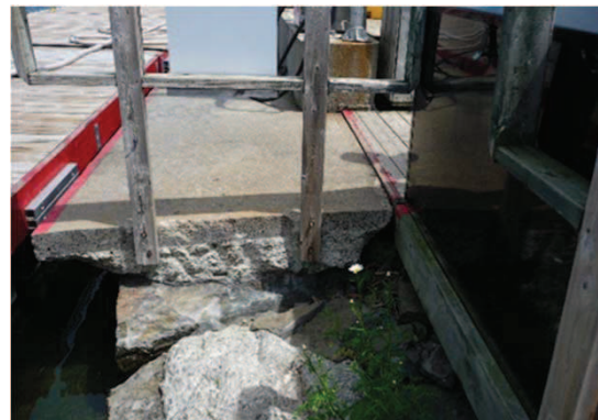
Deterioration of the Marina's service building including the gas station
