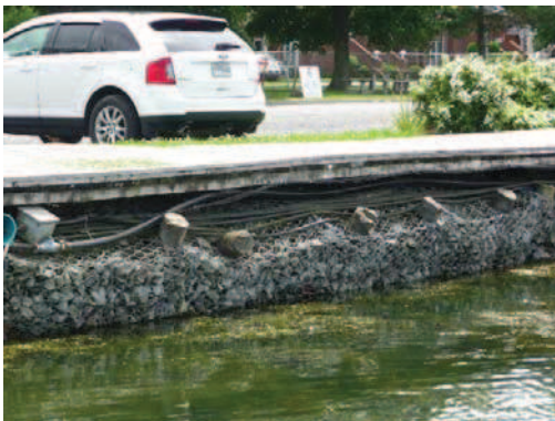
Deterioration of the retaining wall
