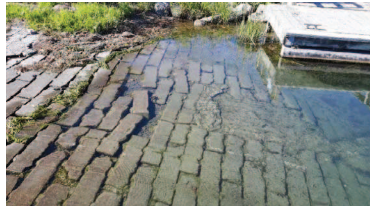
Deterioration of the surface of the existing boat ramp
