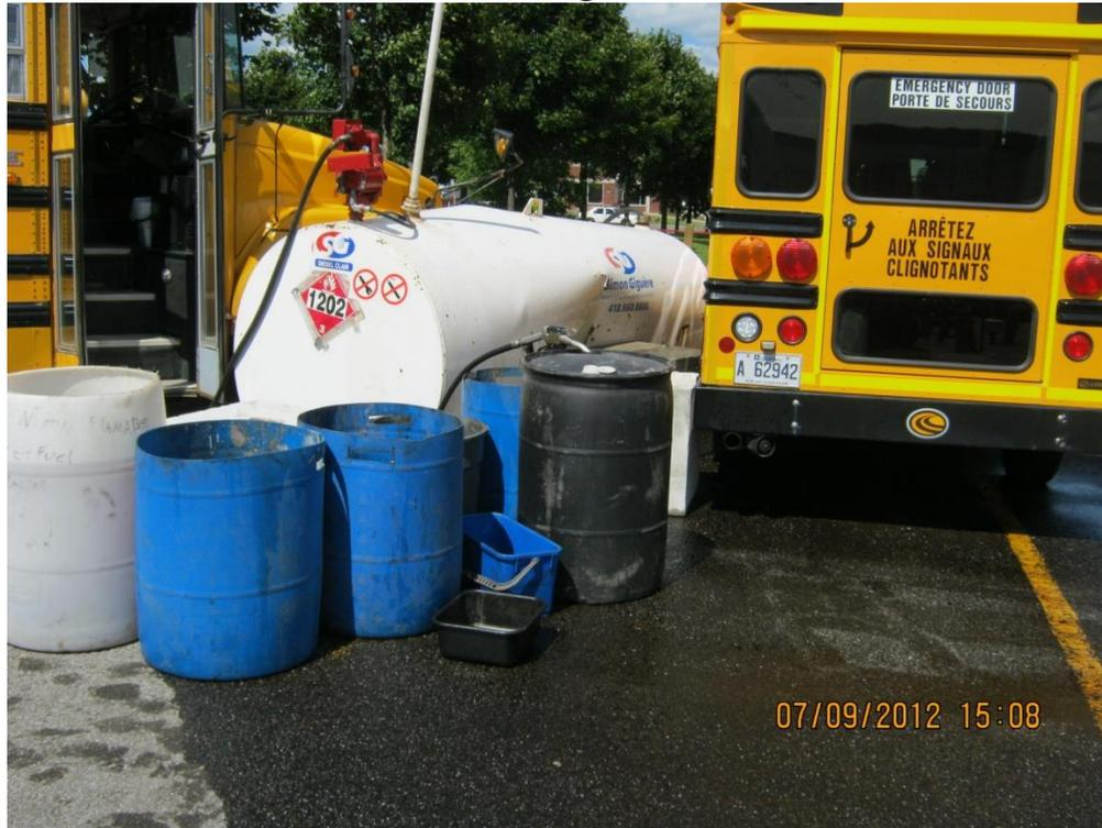
Figure 1 LIEU DE L'INCIDENT. BLOC DE BÉTON POUR PROTÉGER LE RÉSERVOIR NON CONFORME SELON LA RÉGLEMENTATION, 2000 LITRES DE DIESEL DANS LE RÉSEAU PLUVIAL
