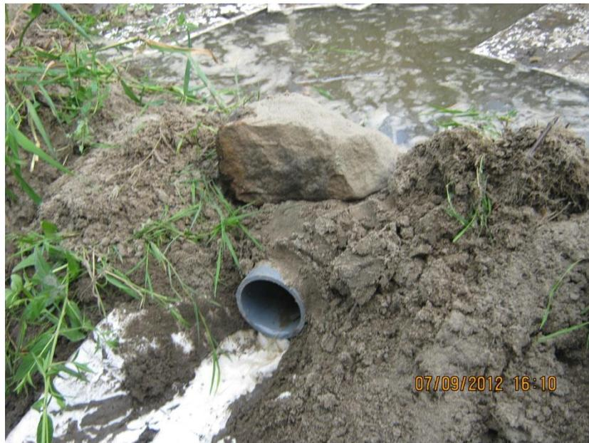
**Figure 4 POSE D'UN DRAIN POUR RECUEILLIR L'EAU PAR LE FOND DE LA FOSSE**
