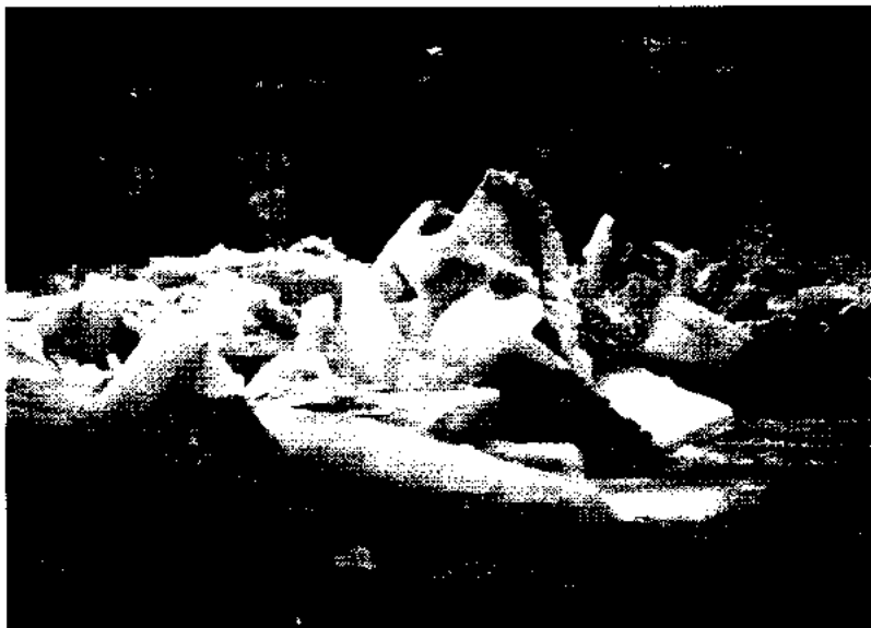
FIG. 15. Ice Pieces Shoved above ICS Blocks during Breakup on March 16, 1995
