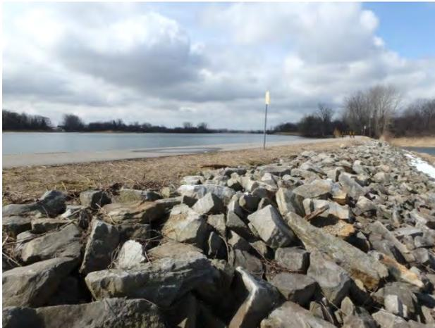
Photo 1 – STRCT 1 – Enrochement in situ 150-600 mm
