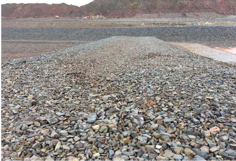
Photo 7 : Water Pond - Internal dyke: differential settlement (mentioned by TSMC in spring/summer 2020) present.
