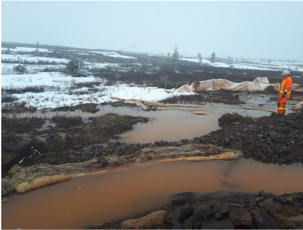
Exfiltration containment structures with filtration socks implemented
