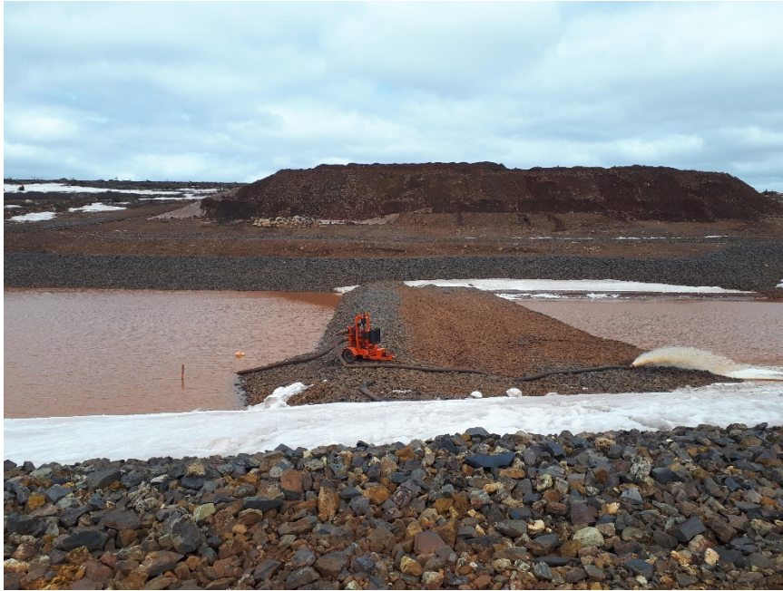
Pumping setup from repair section of pond to temporary containment section
