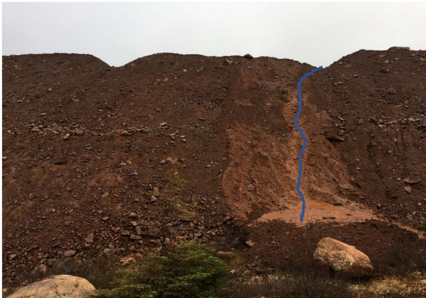
Photo 1 : Overburden Stockpiles - Observations of rilling surface erosion caused by runoff
