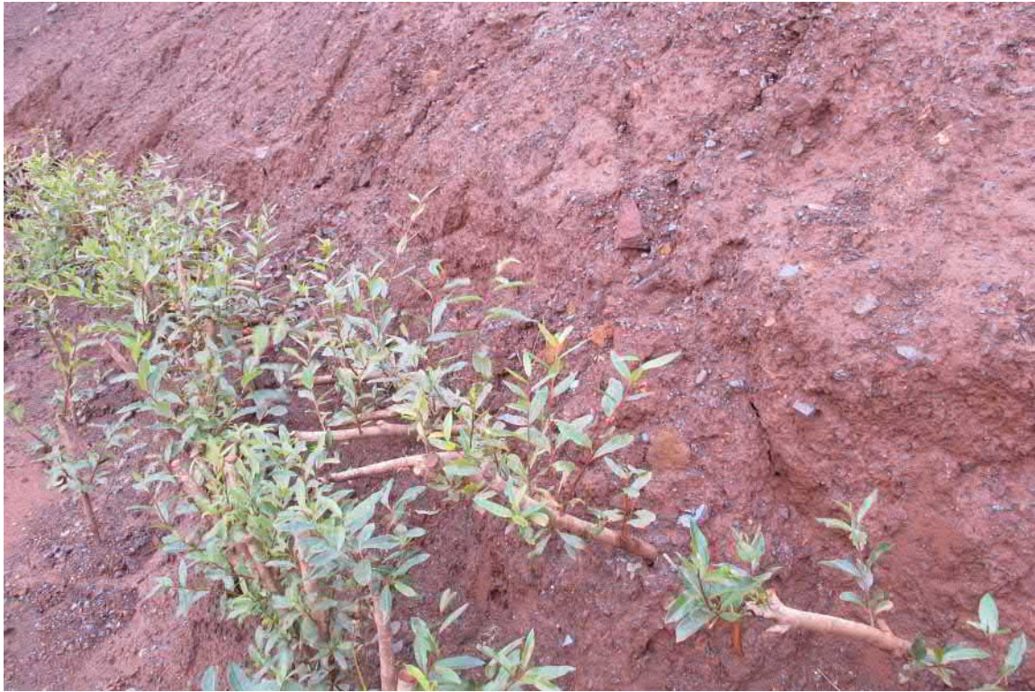
Planeleaf willow large cuttings (60 cm) planted horizontally and vertically for the slope stabilization small scale trial
