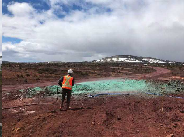
Hydroseeding an experimental block plot
