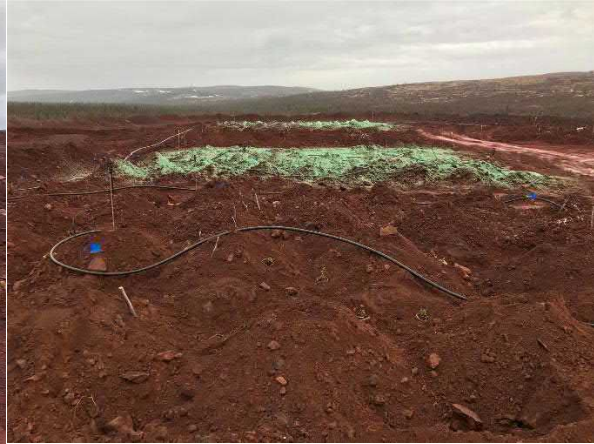
Overall view of the restoration block 1
