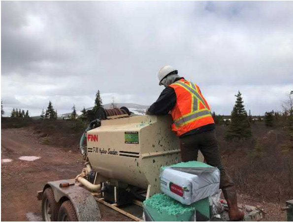
Hydroseeding mix preparation
