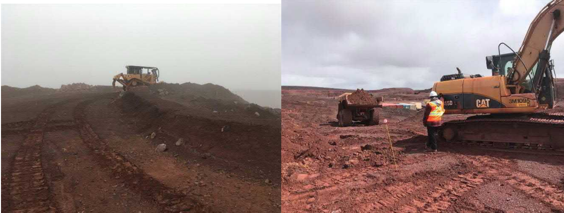
Timmins 4 waste dump slope reshaping Overburden added over rough and loose plot
