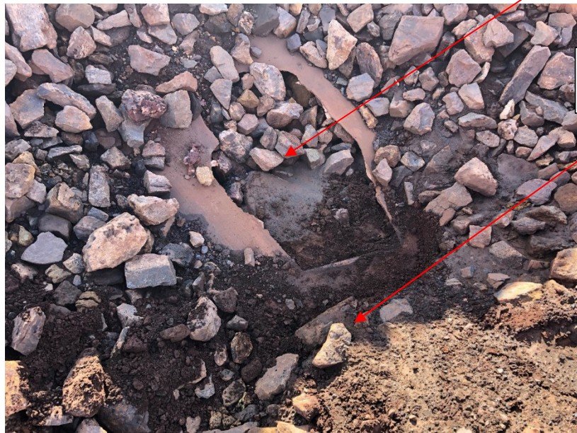
b) HOLE # 1 : The geomembrane is folded into the dike, at the base of the hole. It's a puncture (movement from top to bottom), may be done by an equipment. The hole has created internal erosion of the dike (under the geomembrane).
