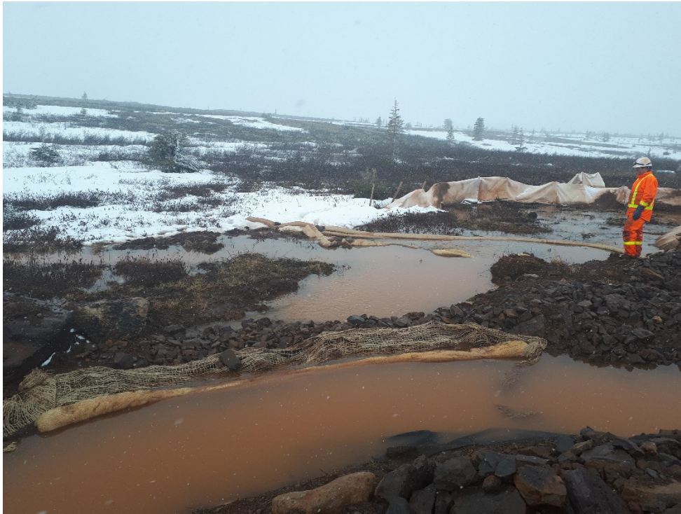
Exfiltration containment structures with filtration socks implemented
