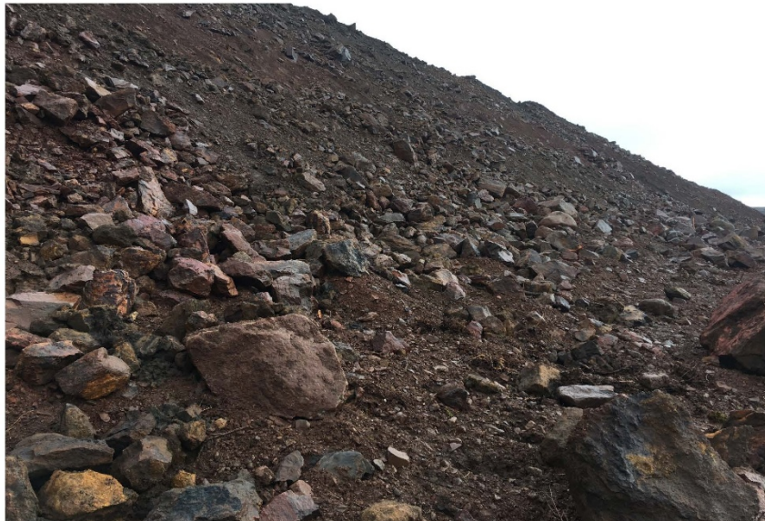
Photo 4 : Active WRD (south-west): material highly variable, from boulder sized particles to soil particles and varying from moderately altered rock to completely weathered rock to soil and silt-like materials
