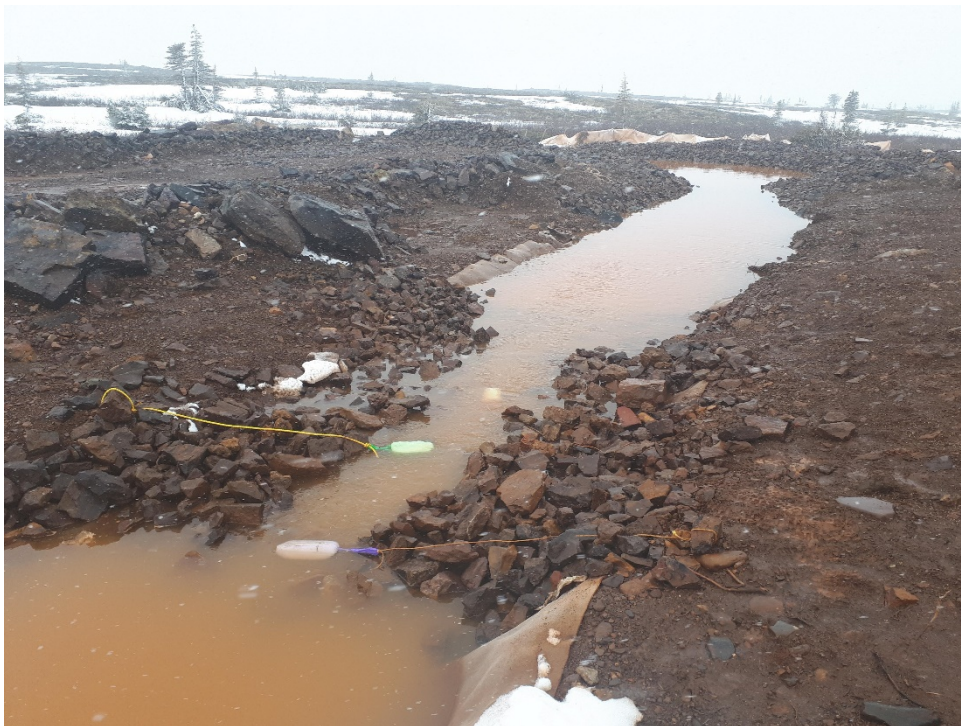
Exfiltration flow looking downstream from toe of dyke; flocculant blocks implemented for clarification
