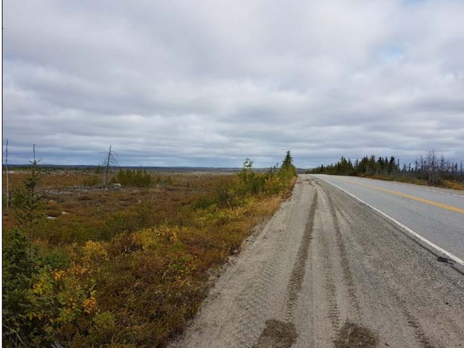
Photo 6-14 Road landscape unit
