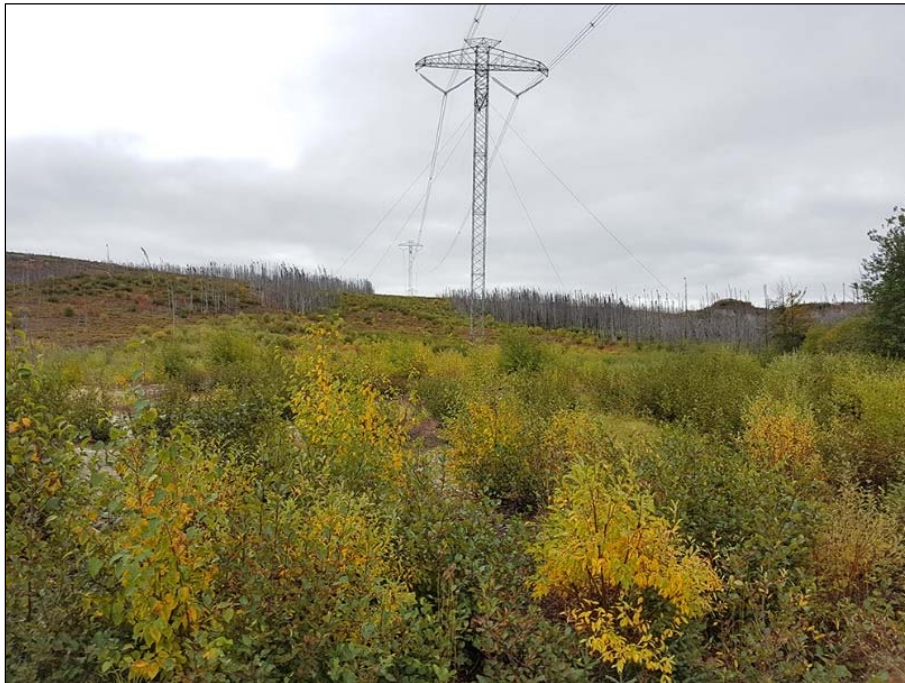
Photo 6-13 Power line landscape unit, view from the Eastmain River valley towards the power transmission equipment
