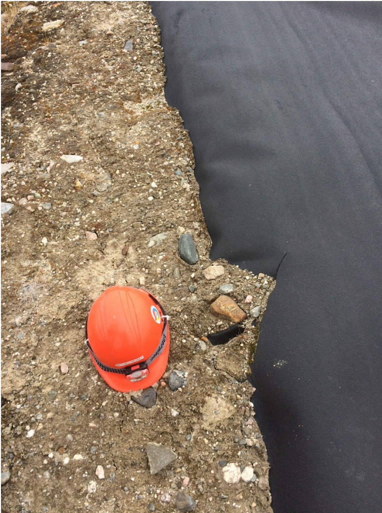
Figure 1 bris membrane
