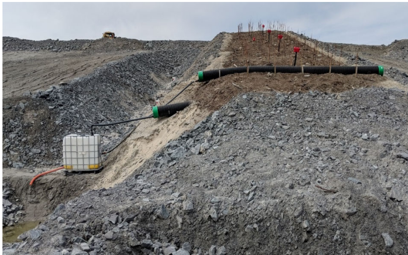
Test pad of the tailings cover
