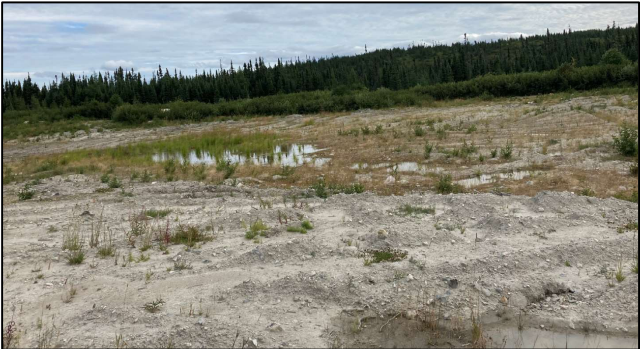
Figure 23: View of the central section with water accumulation (2020-08-29)
