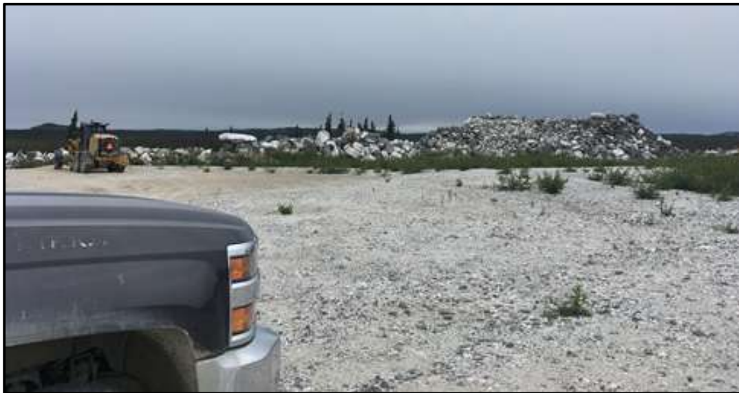
Figure 20: Blasted material pile (2019-07-10)
