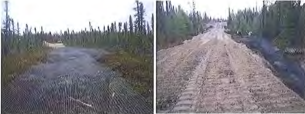
Figure 6 - Example of backfill on geogrid (CA request of November 26, 2012)
