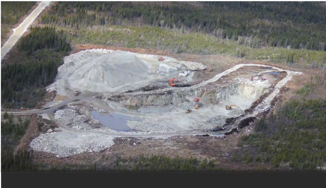
Figure 13 - C-05 quarry in full operation in 2012
