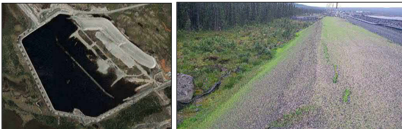
Photo 1 & 2. Typical earth built dykes and slopes around Digue D1. Growth taking place after 1 week of Hydroseed application.
