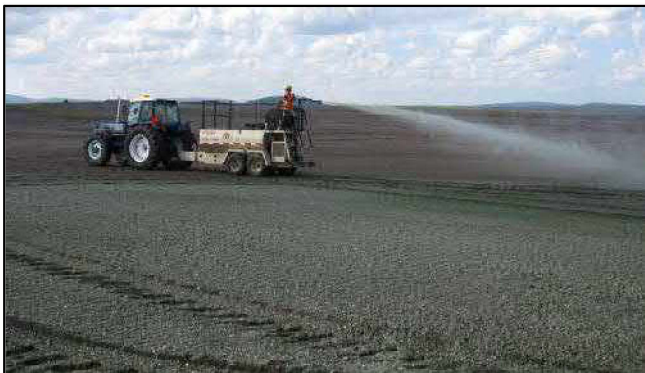
Photos 3&4. Hydroseeding/mulching application.
