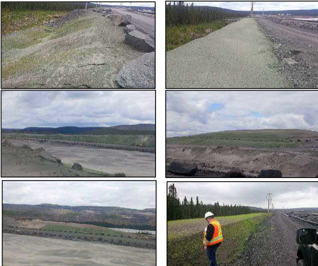
Photos 5, 6, 7, 8 & 9. Various Hydroseeded Areas
