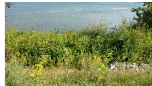
Photo: 66 Berge (type 4) Aucune intervention (1+880)
