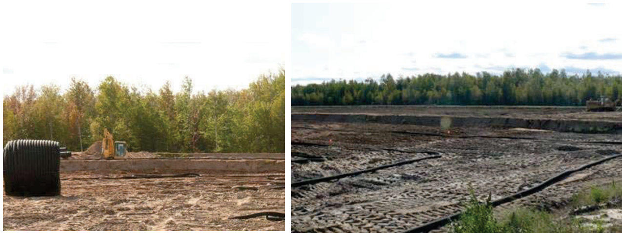
Figure 7. Installation des drains
